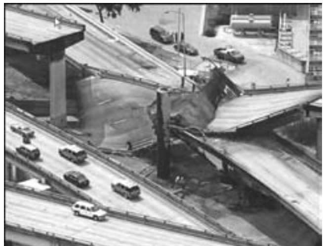
Figure 6. The San Francisco - Oakland Bay Bridge in Oakland, California, 2007
